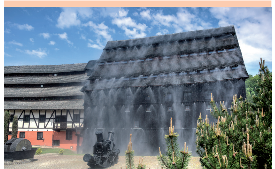
Commissioning of water mist extinguishing system, 2017
