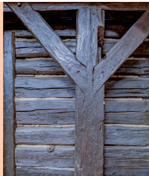
Half-timbered wall in the drying loft, built of logs cut in the 16th/17th century
